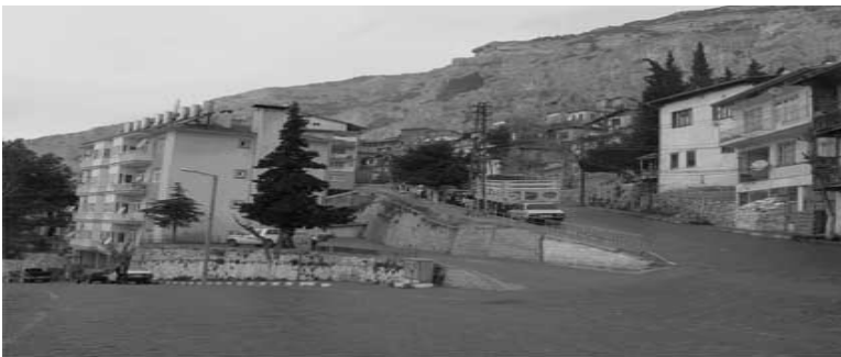
Photograph 3. which cannot be articulated and interpreted in the old and new urban fabric
