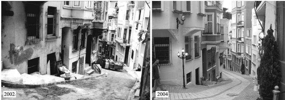
Figure 4. Before and After Adaptive Reuse
