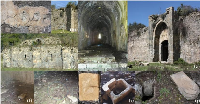
Figure 8. Values in building scale; plaster mason signature (a), triangular buttress (b), relieving vault in shelter roof (c) platform design (d), south facade with different stone usage and portal design (e), latrine design (f), room with *tandır* remain (g), authentic roof tile (h), *yemlik* remain (i), illumination hole with closing stone (j)
