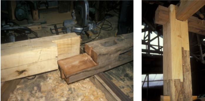
Figure 1. Oyama Dera realized the repair of the elements with partial intervention in the load-bearing elements of the burning pagoda. He developed a detail that ensures interlocking at the joints (Larsen, Marstein, 2016).
