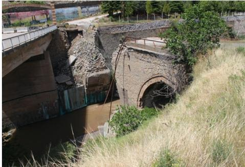
Figure 7. Elazığ-Maden Bridge, part of which was destroyed due to flood and overflow (Authors archive, 2023)
